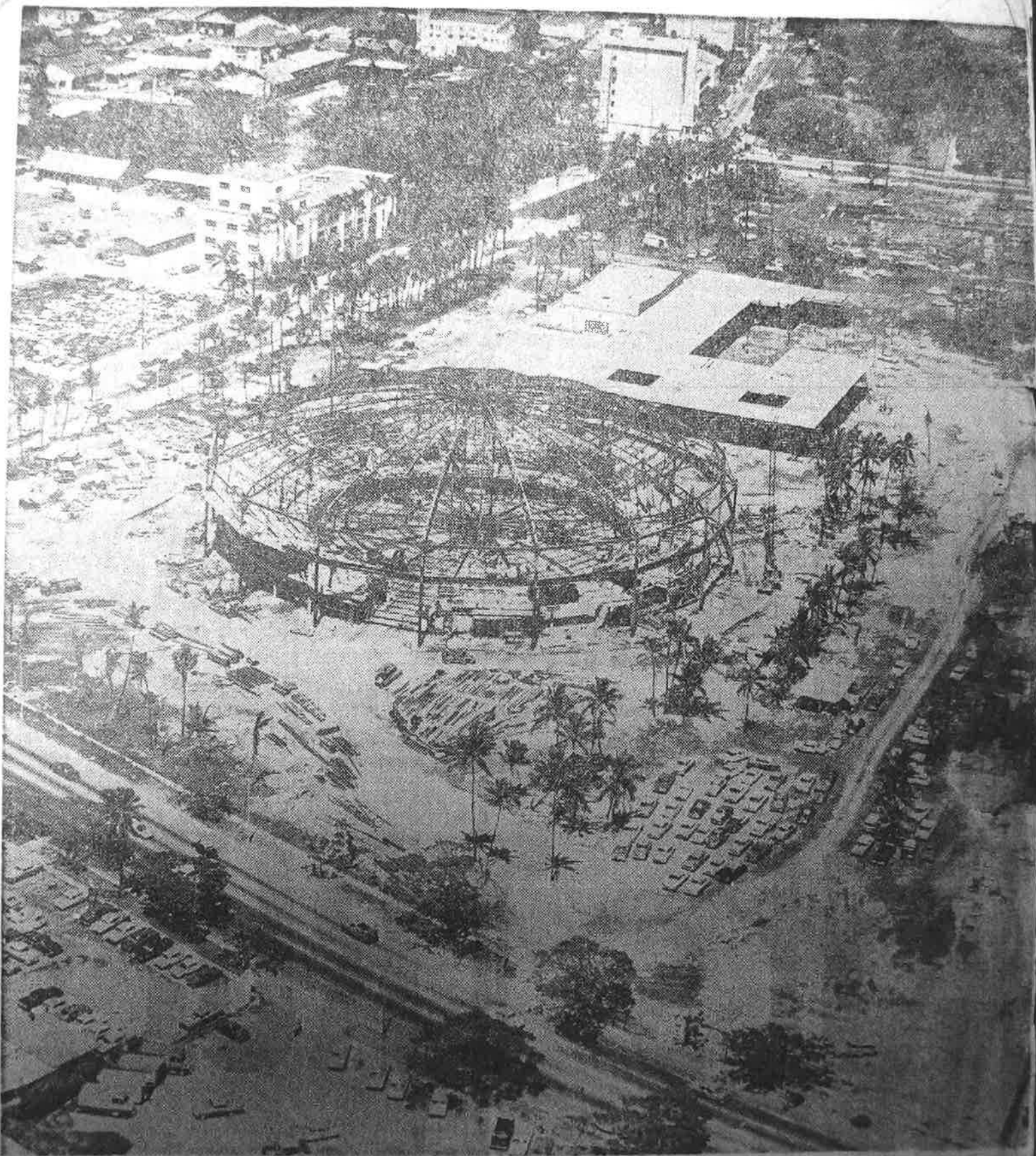
The sports arena of Honolulu's War Memorial Auditorium complex is taking shape rapidly under its canopy of steel girders, which will eventually be covered. In this aerial photograph Kapiolani Boulevard is in the foreground with Ward Avenue at left of the old Ward Estate. Groundbreaking ceremonies were held on May 25, 1962, and the whole complex is scheduled for completion early in 1964. Behind the arena are convention facilities (the building with flat roofs) and a theatre-concert hall is under construction in the background. The arena will seat 9,000 people.—Photo Hawaii Photo.
